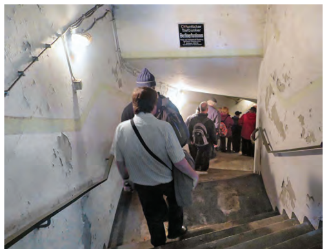
Descending into the three-level Berliner Tor bunker. Luminous paint which parallels the handrails some distance above can just be made out
